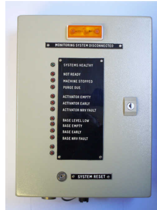
Figure 2: Wall mounted monitoring unit - front view
